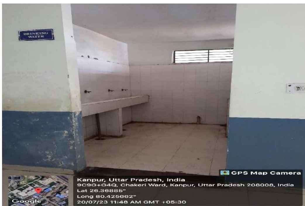
Water Drinking Area 2
