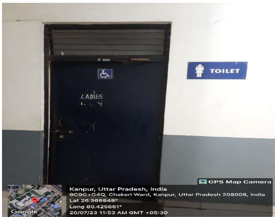
Female Washroom (Differentially Abled)
