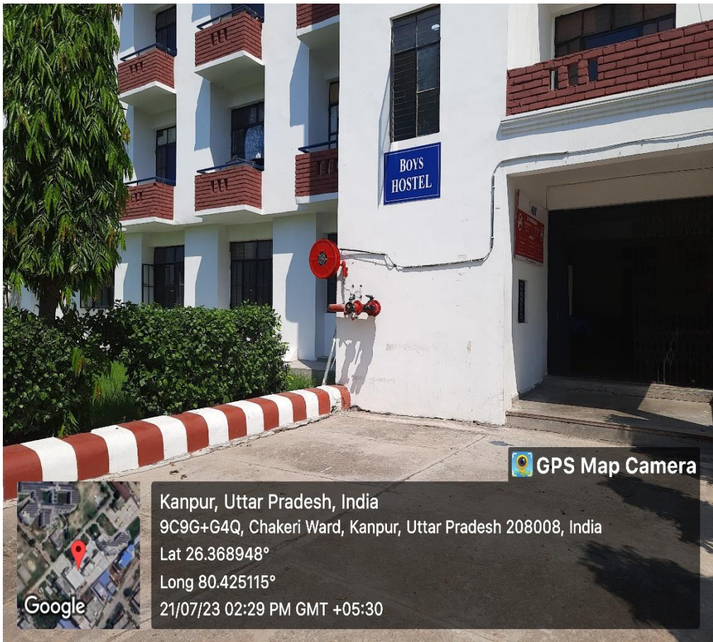
Fire Safety System 3 (Boys Hostel)
