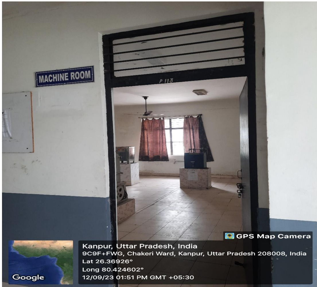
Lab 5 (a): Machine Room
