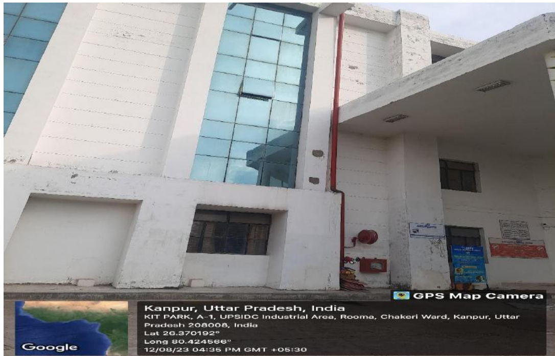
Fire safety System 2 (Academic Block)
