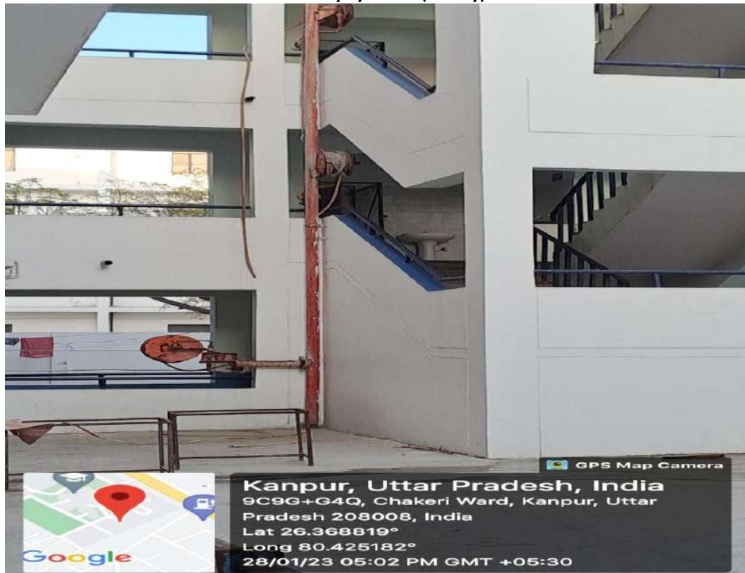
Fire Safety System 6 (Boys Hostel)
