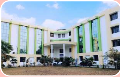
Pharmacy Main Building
